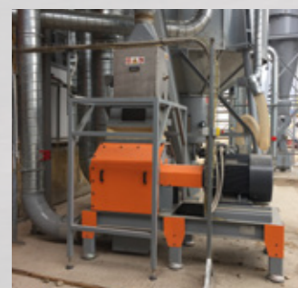
RP03 installato - installed.
